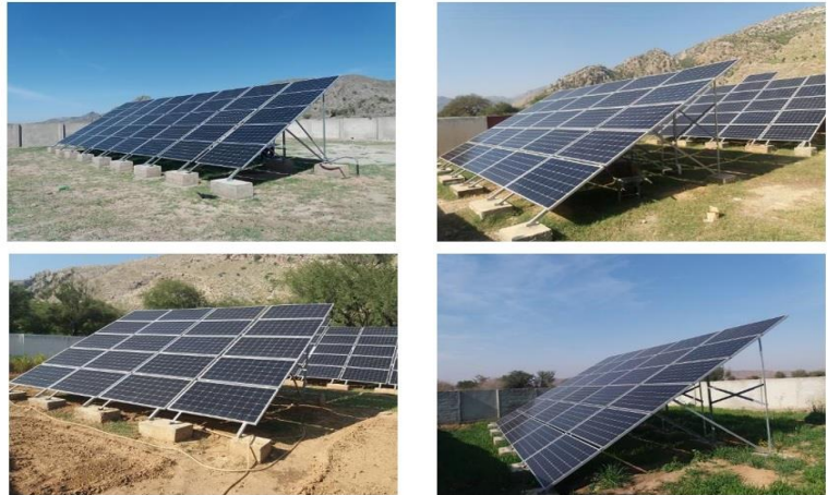
Solar Pumping Projects at FATA Newly merged Area
